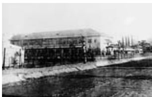
New laboratory of Okayama Plant
