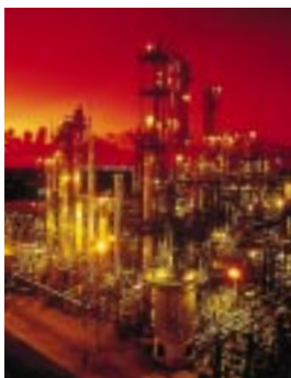
EVAL Company of America, Pasadena Plant
