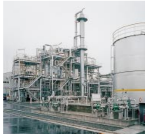
"Kuralon K-II" production facility at the Okayama Plant
