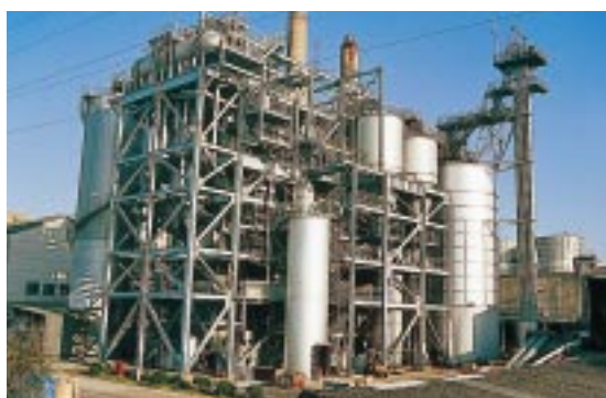
This facility at the Tamashima Plant (Okayama Prefecture) recovers heat energy from waste, such as plastic.
