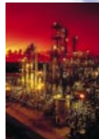
EVAL Company of America, Pasadena Plant
