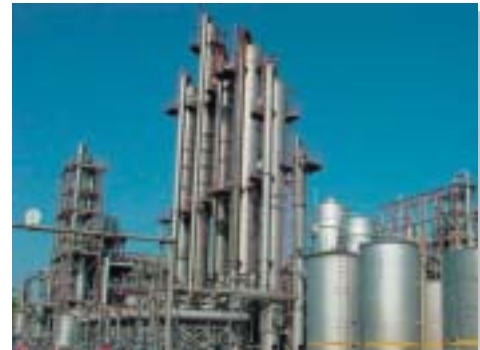
High-pressure Gas Equipment
